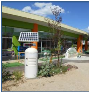
Installation of equipment for measuring radiation
